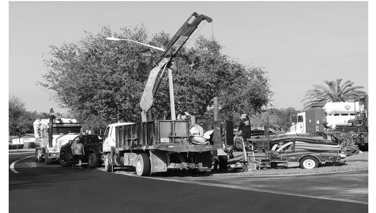
Pipe relining project near Palmetto/Philodendron.
